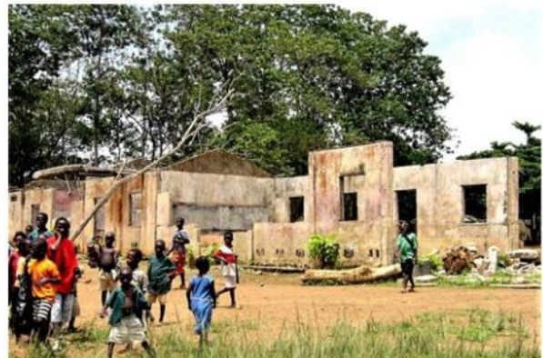
Sierra Leon Civil War : Destroyed school in Koindu. 1991 – 2002
